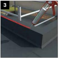
Apply a generous, continuous bead of silicone to the outer perimeter of the top surface of the kerb.
