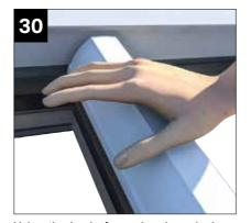
Using the heel of your hand, push down on the top cap to engage the clips, working from ridge to eaves. Ensure the rubber gaskets are fully compressed for a watertight seal. NOTE: on longer bars it may be necessary to use a soft mallet and timber block.
