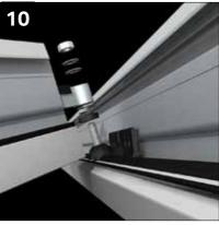
Now fit the jack rafters. The 2 part jack rafter kit is already fitted to the hip and jack rafter. Ease back the jack rafter undercladding. Each jack rafter kit is supplied with a number of washers. Trial fit the jack rafter and check that the glazing platforms are level. Adjust if necessary by adding or removing washers between the two part connecting kit, then tighten the nut. NOTE: If aluminium internal claddings are being used, fit hip internal cladding prior to fitting jack rafters.
