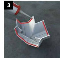
Apply 2 generous beads of sealant to the underside of the external cover.
