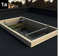
Construct the upstand to the flat roof with minimum of 150mm tall kerb (minimum of 70mm wide). Check that kerb is square by measuring diagonals. Apply membrane as per manufacturers guidelines.
