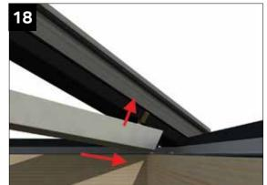
At eaves, slide undercladding down towards eaves as far as you can and push onto clips. Hip claddings are asymmetric. Fit with short cut between hips as shown, claddings have red and blue coloured dots attached to indicate position - always use a red and blue dot at each ridge end.
