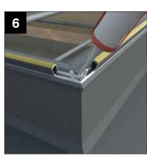
Once eaves beam/rail is fitted, silicone corner joints.
