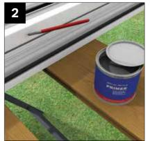
Ensure the surface is dry - apply a thin primer coat using a fine brush.
