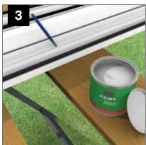
Finally, apply an air drying top coat with a fine brush.
