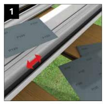
If surface damage is encountered, use 120-360 grit paper to prepare the surface. Wipe clean with white spirit.
