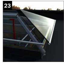
Lift glass units into place onto the glazing bars. When fitting units along the ridge, lift the unit slightly and push into the ridge, then lower onto the eaves glazing support. Centralise the glazing between the glazing bars. If necessary, pack out on each side.
