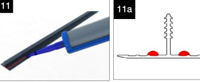
Run a bead of appropriate sealant ensuring a continuous run along the external lower muntin bar. Please see cross section for bead positioning.
