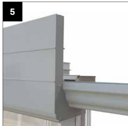
5 CORNICE & FLY THROUGH GUTTER DETAIL - Used when the gutter extends beyond the Cornice. Take the end plate and cut to the shape of the gutter that projects beyond the Cornice.
