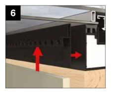
Plasterboard trim fitting - **OPTION ONE** - Fit to edge of plasterboard and then fix plasterboard appropriately
