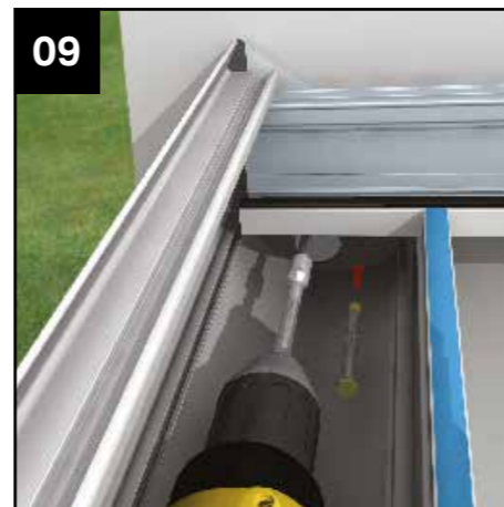
09 Ensure the starter bars are secured to the host walls at each side.
