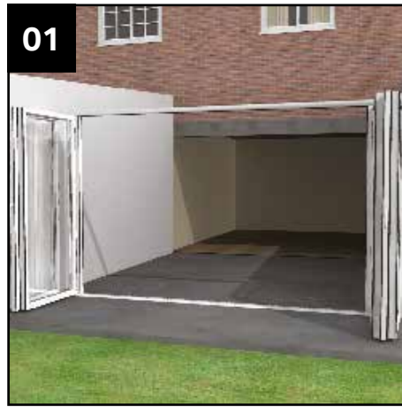
01 Your Veranda construction should look like this prior to roof installation.
