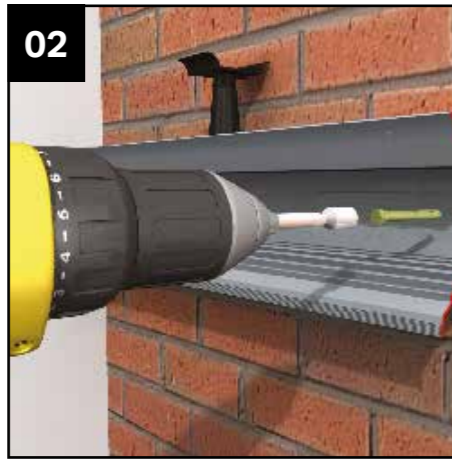
02 Separate the two parts of the aluminium half ridge body. Offer up the main half ridge body which fits between the two side walls. To set the height of the wall plate use the paperwork supplied. Attach to the host wall using anchor bolts at 500mm centres.
