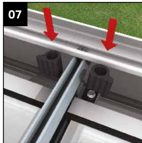
07 Complete the installation of the glass support clips (the clips fit higher than normal).
