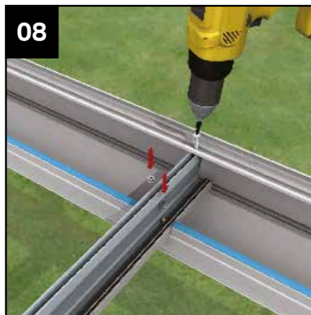
08 Offer up the Veranda beam and secure the roofing bolts with nuts and use the self tapping screws to fasten the leading edge of the veranda beam into the head of the aluminium glazing bars using CRN010 fixings.
