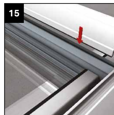
15 Complete the installation of the cappings.
