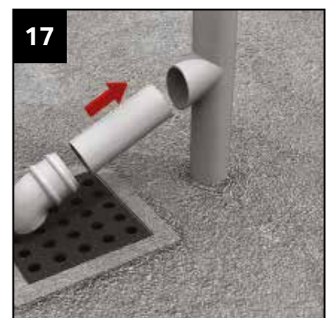
17 If required, cut supplied rainwater downpipe to length and attach downpipe shoe. NOTE: A footplate is sent out as standard.
