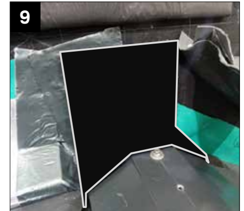
Fit the supplied host wall flashing cap using a low modulus silicone.
