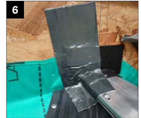
Image shows examples where 1 Butyl patch is applied - Glazing on duo-pitch segment (main image) and glazing on lean-to segment (inset image)
