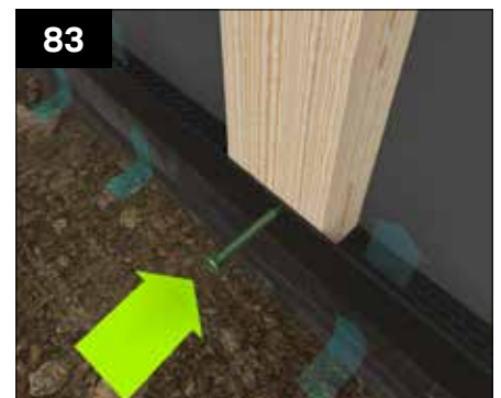
At the base of the wall attach the perforated ventilation trim to the battens. This allows for ventilation and drainage but inhibits vermin/ insects.
