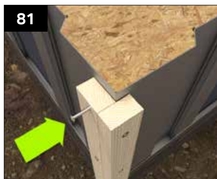
At corners battens should be fixed as shown. This ensures that wall finishes (claddings) at the corners are well reinforced.
