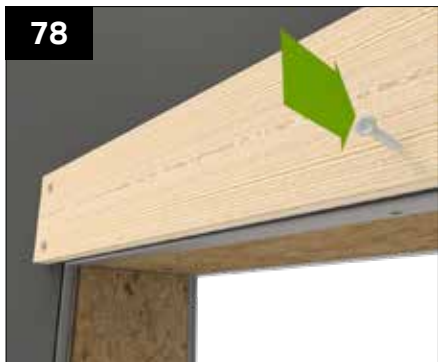
Above openings, fit a horizontal batten across the top of the opening at 450mm centres with the base of the batten aligned with the opening in the wall.
