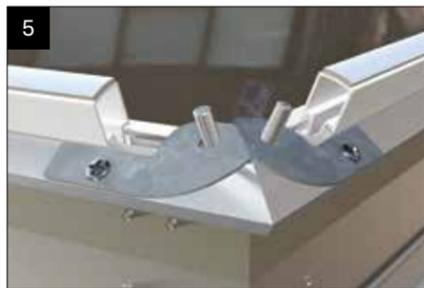
5 An additional cleat is inserted in the eaves beam corners (making two cleats in total) whilst this is backed up by a further butterfly cleat (illustrated).
