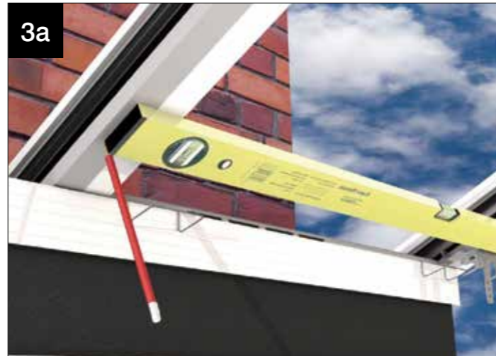
3a FITTER TIP: If possible, check and line through with the bracket position on the adjacent full length bar. Mark the bracket positions on the bars off the box gutter.
