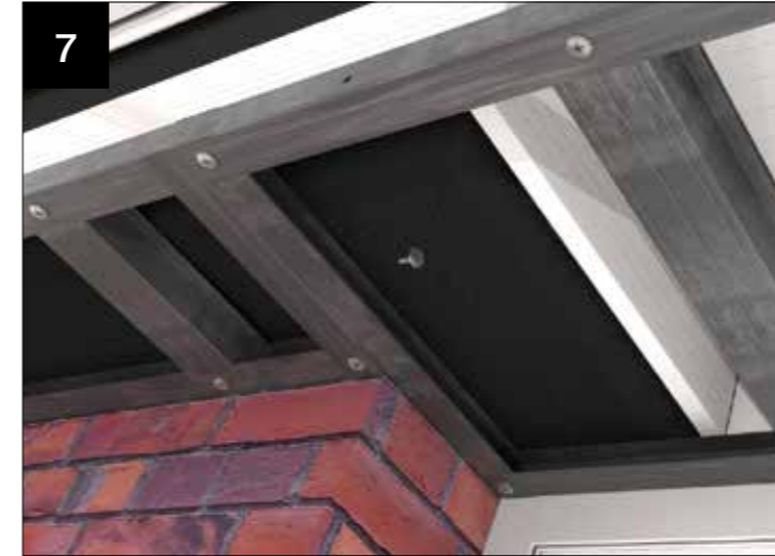
7 Screw split horizontal frames together using CHAA006 (bag of 25).
