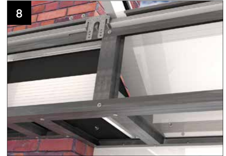
8 Fix the vertical frames in place using CHAA006 (bag of 25) as per standard installation.
