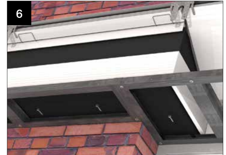
6 Fit back horizontal frame using CHA008 (bag of 25) as per standard installation.
