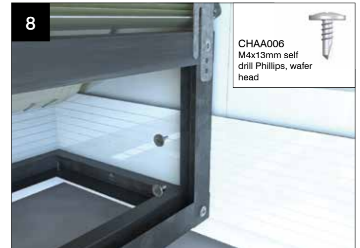
8 Fix the vertical frame into the fascia board using 2x CHAA006 (M4 x 13mm) self drill Phillips, wafer head screws (supplied).
