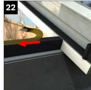
Peel back a small tab of the protective film on the glazing support from the eaves and the ridge. (ready to be pulled away when the sealed units are finally in position). **DO NOT FULLY REMOVE TAPE YET.**
