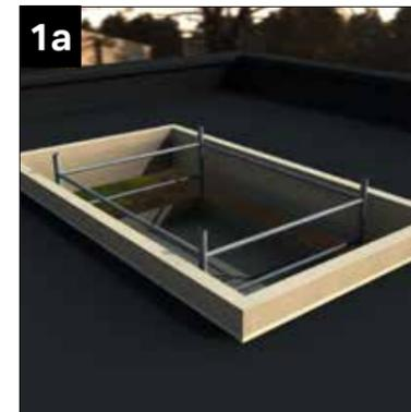
Construct the upstand to the flat roof with minimum of 150mm tall kerb (minimum of 70mm wide). Check that kerb is square by measuring diagonals. Apply membrane as per manufacturers guidelines. The customer must ensure that the kerb and surrounding roof can adequately resist the horizontal spread of the lantern.
