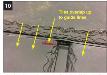
When inserting next layer, overlay tiles in line with insertion lines (marked in red above) on the tile. Repeat steps 8, 9 and 10 until the roof is fully tiled. See tile finishing references on back for accurate fit and best results.
