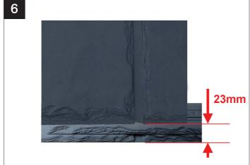
Using the tile location plan provided, locate position of first tile panel (labelled aa1), slide down onto the starter strip leaving 23mm from the starter strip edge. This allows expansion of the tiles in warm temperatures.
