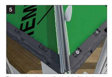
This image shows the starter tile strips being fitted to the already marked hip spine lines (the hip spine will have been removed).
