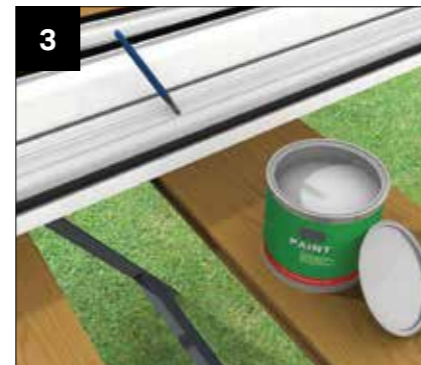
Finally, apply an air drying top coat with a fine brush.
