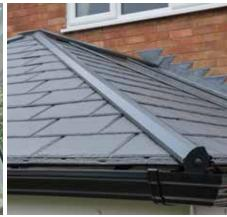
Ultraroof offers a magnificent vaulted plastered ceiling on the inside enhancing the feeling of space within your current conservatory. Thermally efficient with a U-Value of 0.15 with option to reduce to 0.13 if required, Ultraroof offers you the warmth and brightness you require, with beautiful and authentic looking lightweight tiles externally, with the option for full height glazing to flood your home with light and create a stunning feature. The lightest tiled roof on the market 38Kg/M2.
