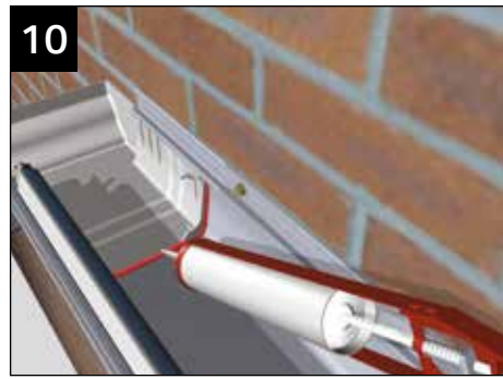
Use the balance of the Gutterbond to back point any gaps at the front edge.
