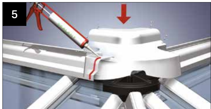
5 Now, as per main guide, seal around each glazing bar top cap where it meets the inner wall of the 'soft touch' weathering shield. Take the length of PVCu ridge top cap assemblies, seal the two ends to be joined. Mark and drill for final rivet positions using a 5mm drill bit. Apply plastic rivets. Offer the whole assembly into position, trimming may be required - see over page. The trimming should be in the form of removing a strip across the whole width or as shown above, notching around each bar. Secure ridge into position with 'T' bolts as shown in section 4.
