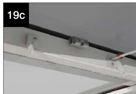
19c Secure the brackets to the frame using screws provided.
