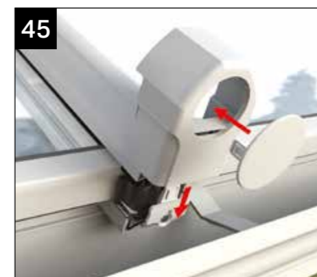
46 If you haven't fitted already, attach end cap fixing blocks - These arrive attached to the end caps. Fit the glazing bar end caps by sliding onto the fixing blocks. Push fit the insert into the end cap.
