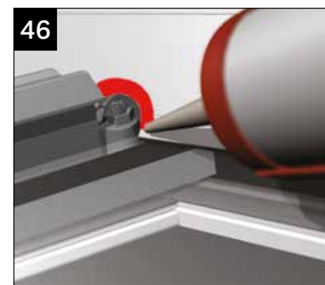
47 Seal around the notched Georgian top cap ready to receive the jack rafter capping.
