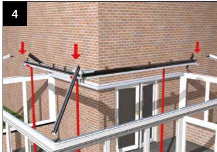
4 Temporary support/prop the 'L' shaped ridge. Offer up the hip bars. Secure using steps 12-15 in the main installation guide. Build remainder of the roof as section 4.
