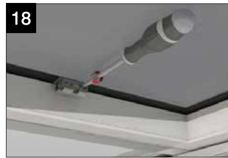
18 Using the nuts and bolts provided attach the motor bracket to the sash bracket taking care not to damage the glazed unit.
