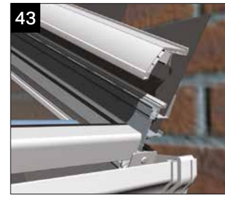
43 Ensure the rain baffle upper leg is lifted prior to fitting the top cappings.
