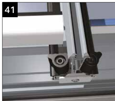
41 Centralise the glazing between the glazing bars. If necessary pack it out on each side - press it down onto the support trim.
