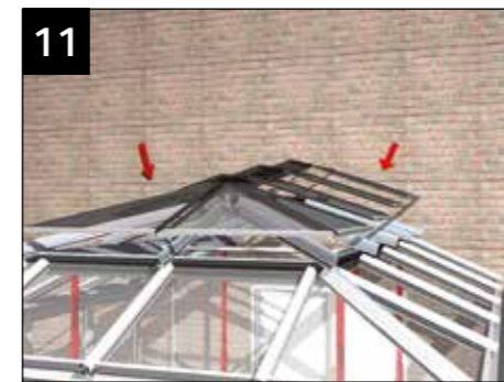
Glaze the upper pagoda roof, and complete all external works
