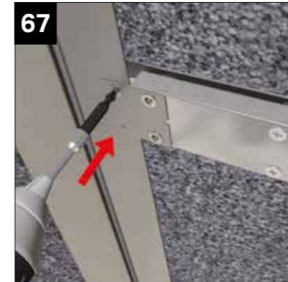
67 Secure attachment plate using 2 x CHAA 006 screws provided to the ridge body.
