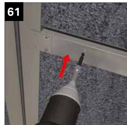
61 Firstly secure into the panel (at the ridge end) using dry wall fixing screws WPDS020 NOTE: See method of alternate tightening as shown 63-65.
