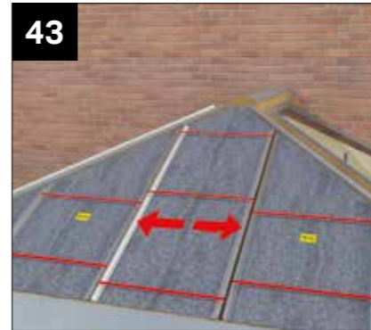
The expandable panel will expand to take up any tolerance gap. Snip the binding cord on all the remaining front facet panels.
