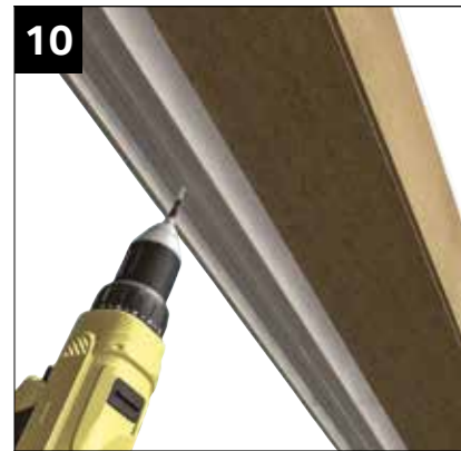
After checking the correct overhang secure the gable panels by screwing up through the head of the frames. Fixings need to be within 200mm of each corner (dependant on access) and at 450mm centres using for example, 4.8mm x 80mm screws; not supplied.
