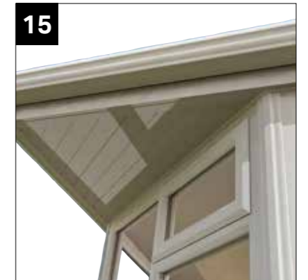
15 Cut and fit ship lap to suit.
