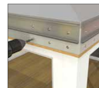
Securing corner cleats
