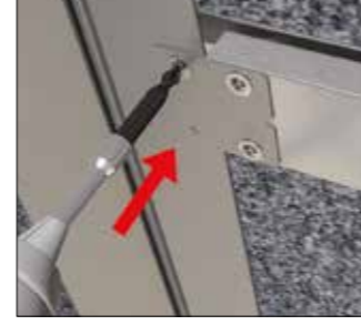
Fixing internal clip to ridge shelf
