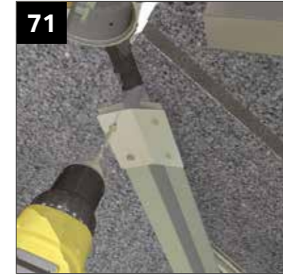
71 Fix the internal upper hip brace plate using 4 x CHAA 006 screws provided.
