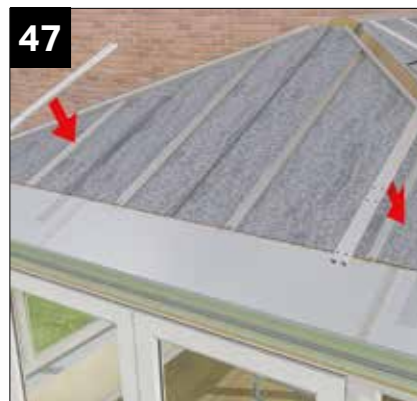
When all panels installed continue to fit the pre drilled external panel clips (see next image for positioning alignment)
