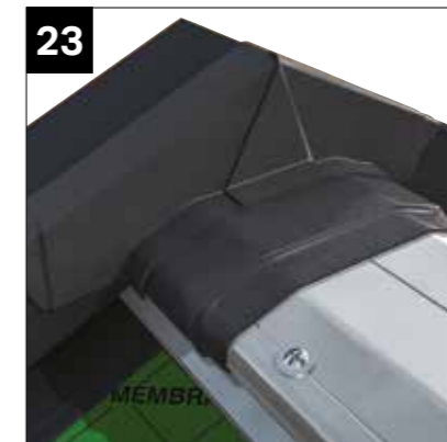
23 Finally cover joint with a third layer.
