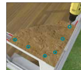
Fixing support shelf to existing frames
