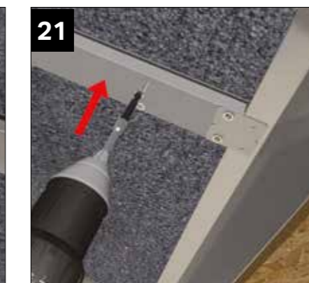
Secure into the panel (at box beam end) as previous image. Again, note method of alternate tightening sequence 22 to 24.
