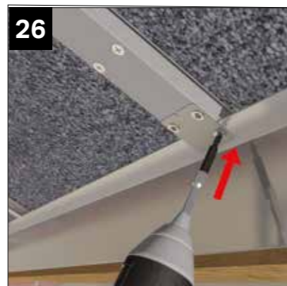
Finally secure to box beam support shelf the lower attachment plate using 2 x CHAA 006 fixings.
