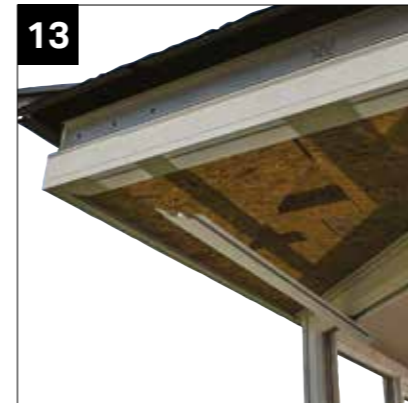
13 Fit external ship lap cladding edge channel.
