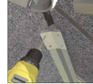
Fixing internal upper hip brace plate
