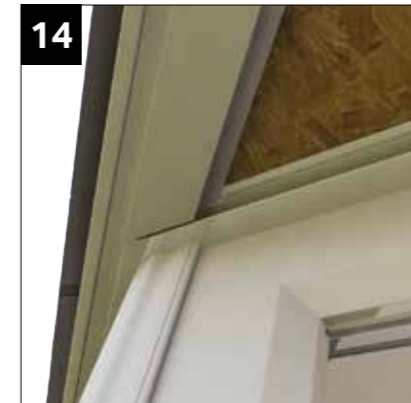
14 External ship lap cladding edge channel detail.
