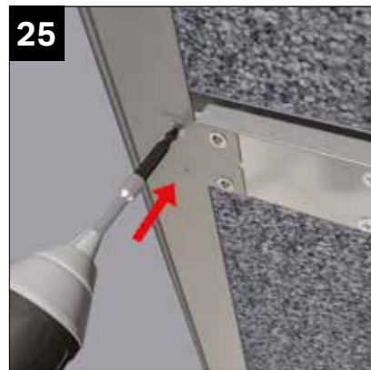
Secure to the half ridge body, the upper attachment plate using 2 x CHAA 006 fixings.
