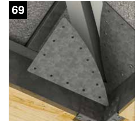
69 Fix the internal hip retaining plates using 18 x CHAA 006 screws provided into the box beam shelf and hip bar. NOTE: These plates are not required on victorian hips.
