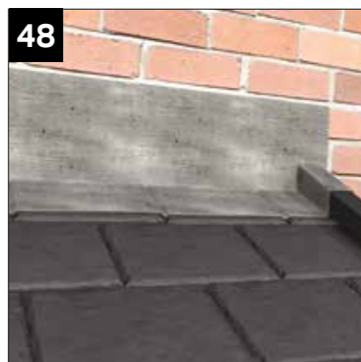
48 Lead flash to existing host wall.
