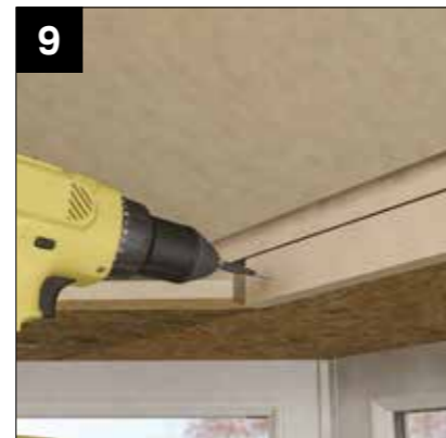
9 Attach additional mating timber battens.
