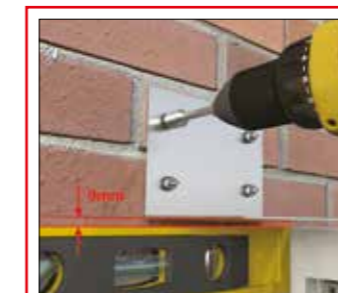
Fixing hanger bracket to wall
