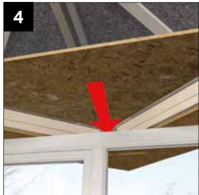
4 Slide into position additional external OSB board.
