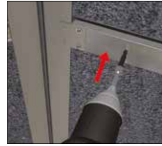
Fixing internal clips
