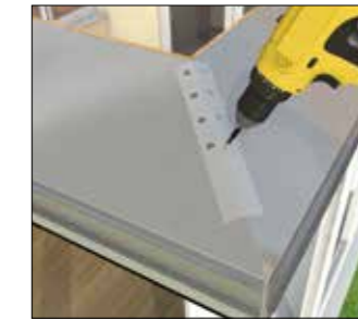
New extended external box beam cleat
