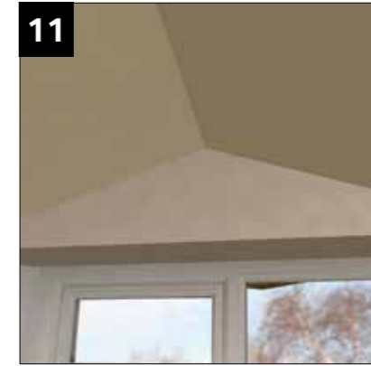
11 Plasterboard face of gable
