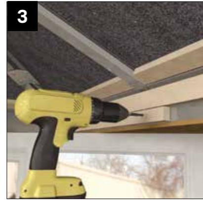
3 Attach additional battens.
