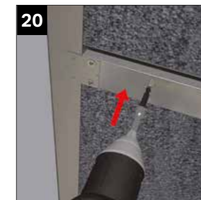
Firstly secure into the panel (at the ridge end) using dry wall fixing screws WPDS020 NOTE: See method of alternate tightening as shown 22 to 24.
