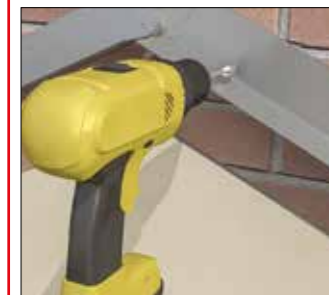
Fixing starter bar extrusions to the wall
