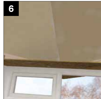
6 Plasterboard the roof.
