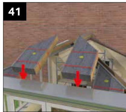
Next, install Ultrapanel working from each hip bar towards the centre.
