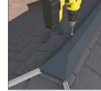
Fixing ridge top cap
