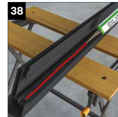
Apply a bead of clear low modulus silicone to the underside of the dry verge.
