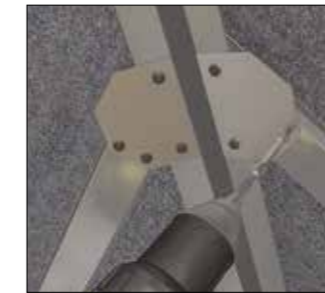
Fixing internal jack rafter connection plate
