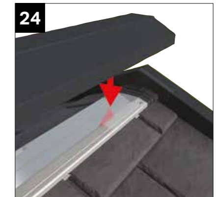
24 Fit the ridge top capping using the NRRSA 005BL supplied.
