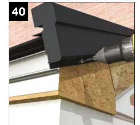
Fix the dry verge to the OSB using NRTS 050 screws at 300mm centres. Ensure membrane overlaps into dry verge for drainage.
