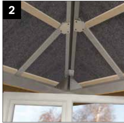
2 Batten out to suit plasterboard fixing.
