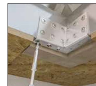
New internal 90° box beam cleat
