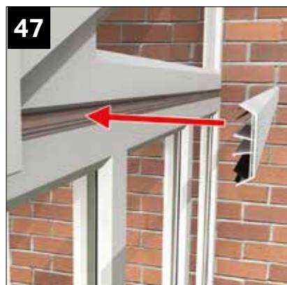
47 Fit internal and external gable stiffener claddings (if ordered). NOTE: Aluminium stiffer and cladding may need notching/ routing for frame drainage.
