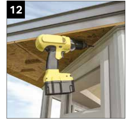
12 Fit external soffit channeling.
