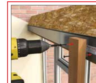
Fixing support props to beam
