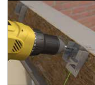
Fixing glazing bar shoes at box beam
