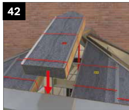
Lower into position the front facet panel. Marked with a red label.
