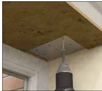
Fixing wall brackets to the beam
