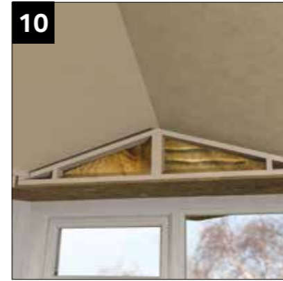
10 Insulate void with mineral wool.
