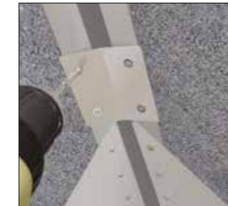
Fixing internal lower hip brace plate
