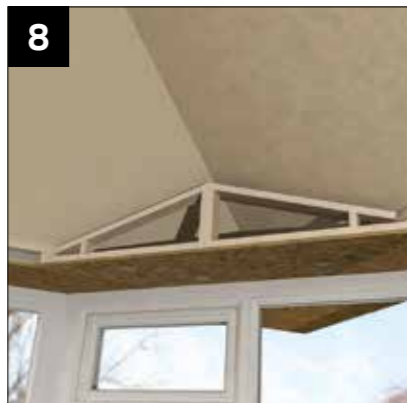
8 Fix into place.
