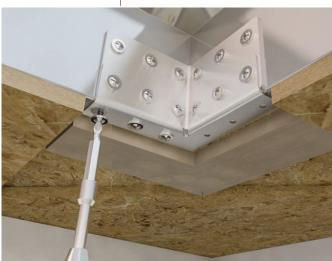
Offer the supplied brackets to the eaves beam as shown and screw fix into position with the 13mm long fixings provided (CHA006). Note that cleat strap WPBBF090 is only required on 90° mitres.
