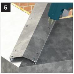
Fix the hip down into the beam through x 4 predrilled holes using WPCS020 (supplied).
