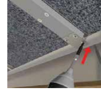
Fixing internal small tab plate to wall angle 2 fixings into wall angle
