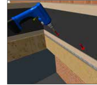
Securing kerb to aperture 1 per 300mm centres
