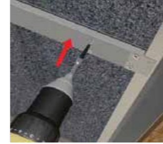
Fixing internal clip to panel 4 fixings per panel
