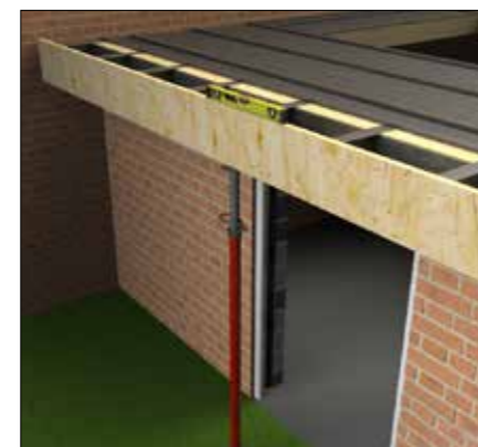
Use a prop to level up the joint before the final fixings.
