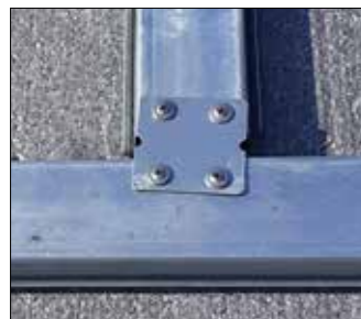
Small tab plate to external panel clip 4 per plate
